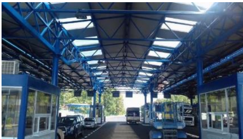
Border Crossing Batrovci (Phase II) (construction completed)
