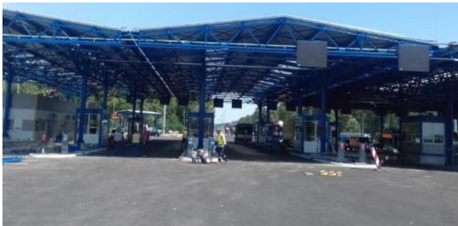
Border Crossing Batrovci (Phase II) (construction completed)
