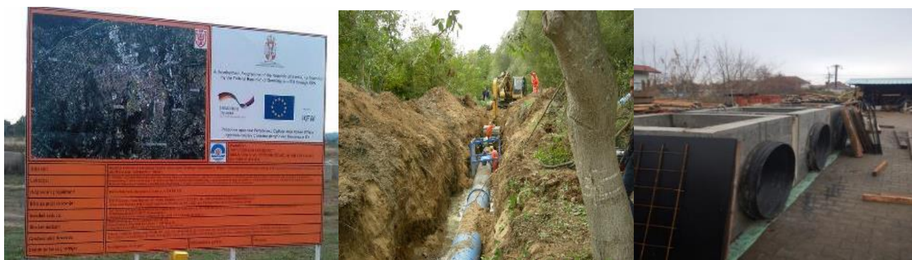
Waste water (WW) collection and WW treatment plants - Krusevac and Vranje (works in progress)
