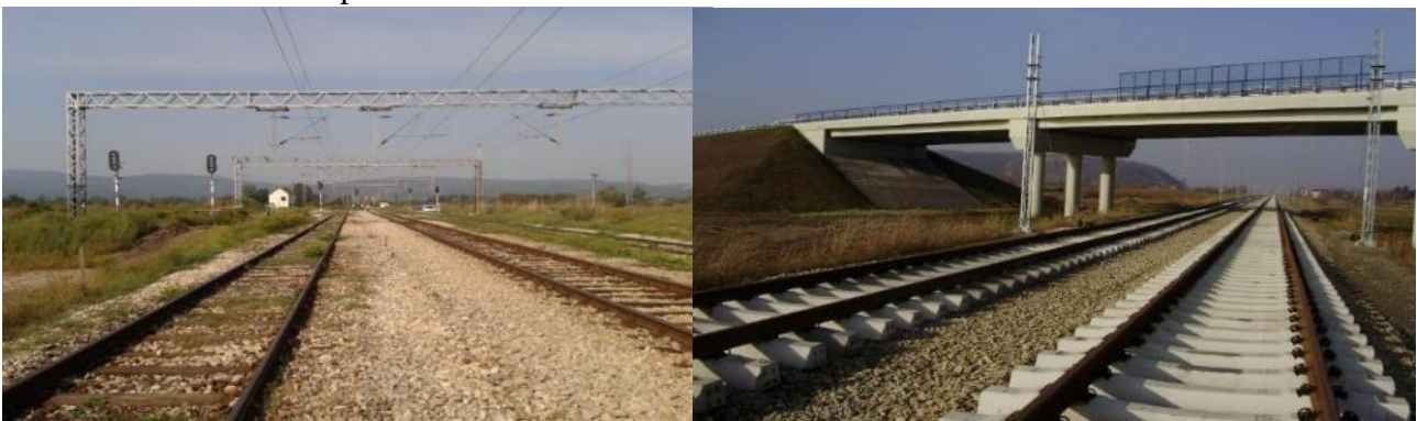
Section: Batajnica to Golubinci (before and after)
