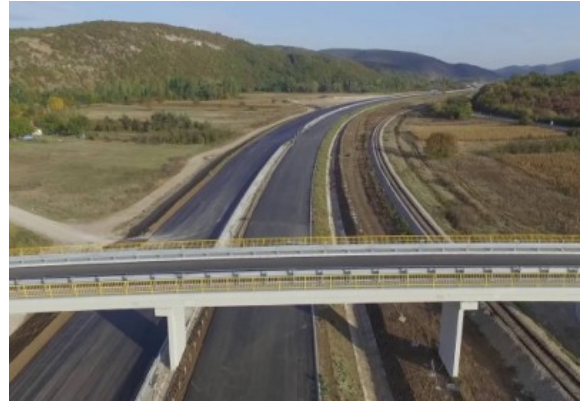
Section: Ub – Lajkovac (construction completed)
