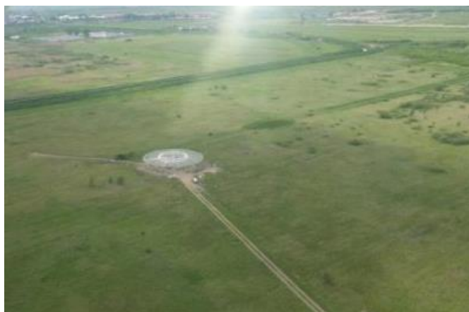
DVOR device at the location of AKL Vršac
