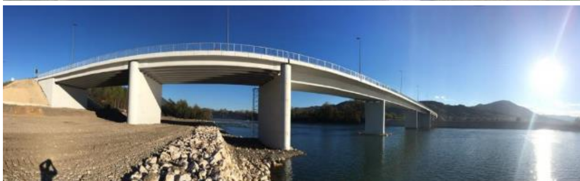
Bridge Ljubovija – Bratunac (before and after)
