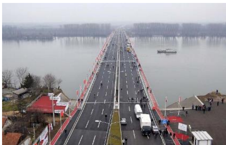
Bridge Zemun – Borca
