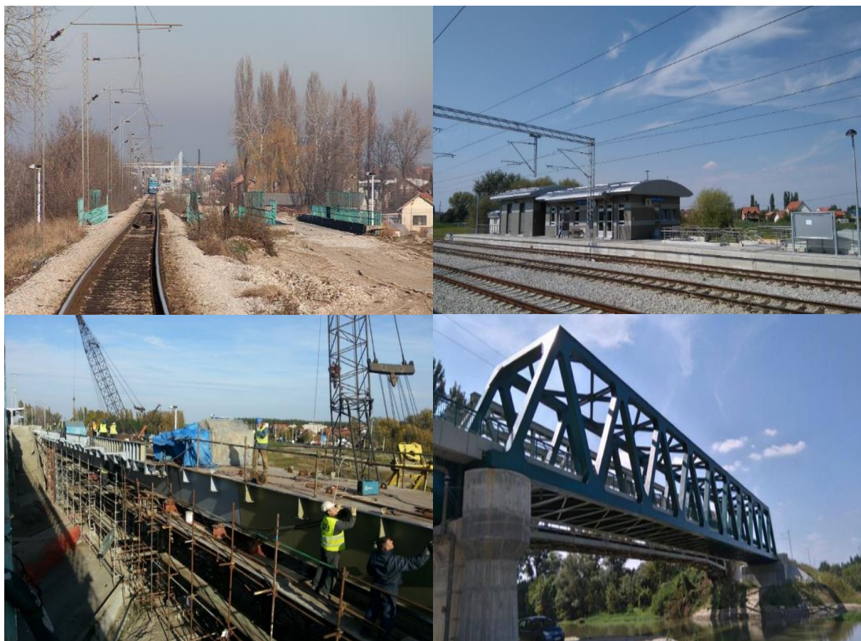
Construction second track of the railway line Pancevo Bridge to Pancevo Main Station (before and after)
