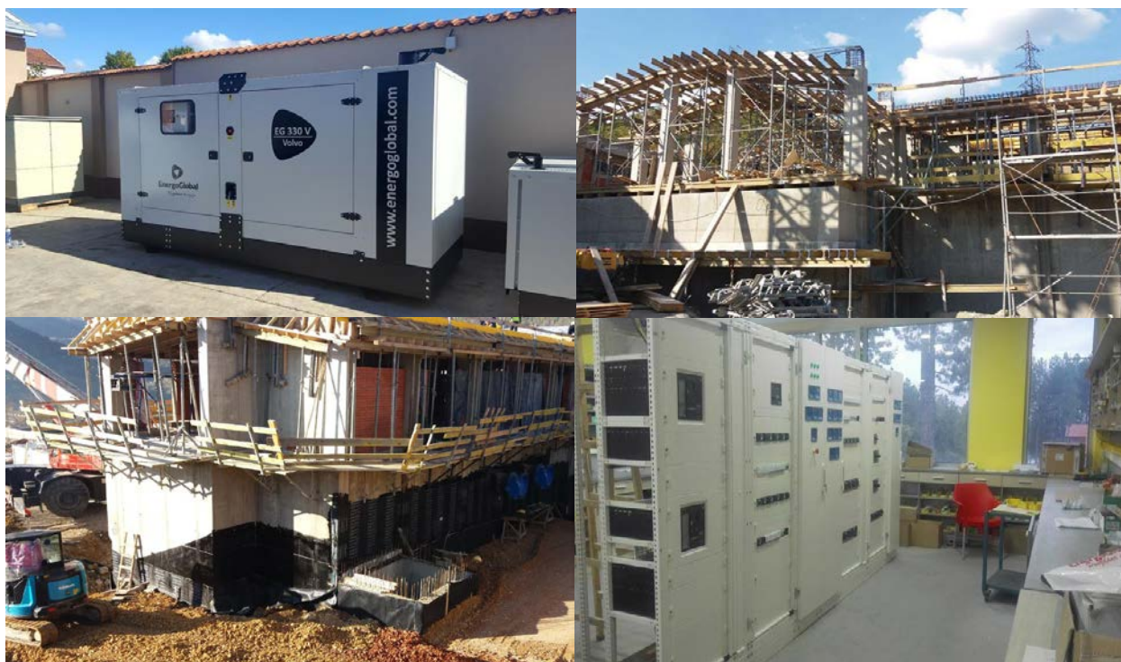
Reconstruction and extension of the effluent treatment plant - Užice (I phase)
