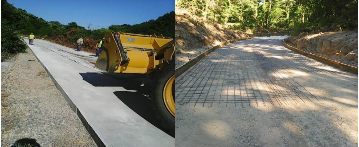
Section: Stara Pazova – Novi Sad (construction in progress)
