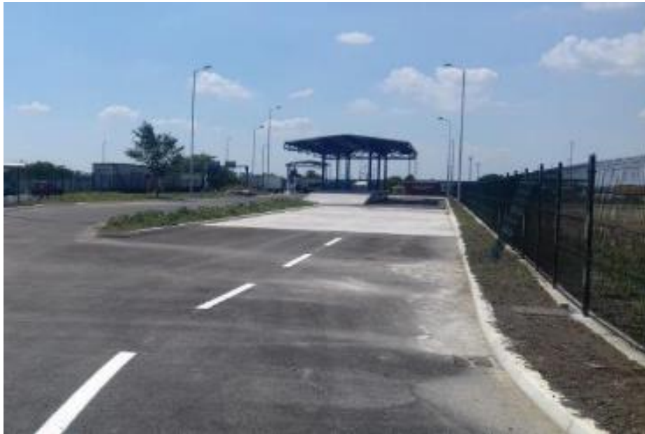
Border Crossing Batrovci (Phase II) (construction completed)
